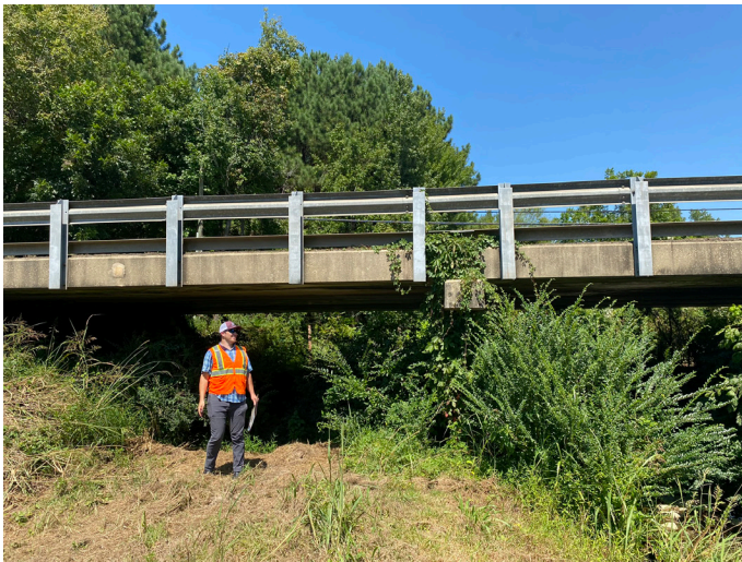
W Balfour Ave bridge at Hasketts Creek
