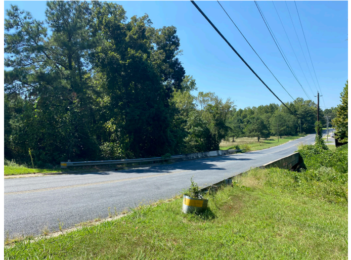
W Bailey St bridge over Hasketts Creek
