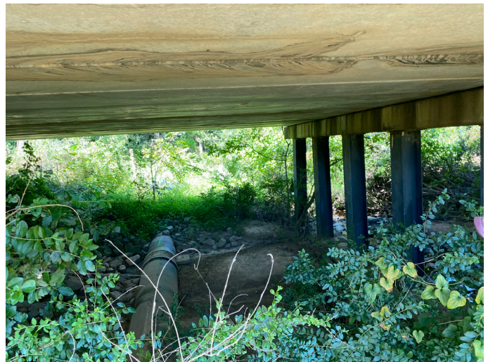
Sewer line under W Balfour Ave bridge
